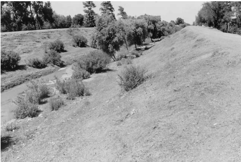
Figure 3.5 Aztec embankment built to contain the new channel of the Cuauhtitlan River in the Valley of Mexico (photograph by William E. Doolittle; reproduced with permission)
