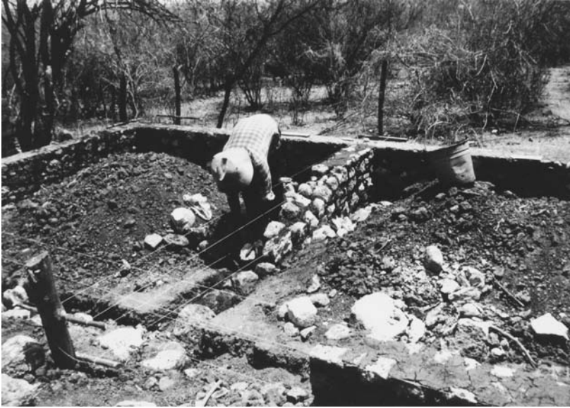
Figure 13.10 A farmer in the village of Tetlama, Morelos, builds the stone foundation for a traditional-style house of adobe bricks. The resulting foundation walls are almost indistinguishable from nearby Aztec peasant house foundations; see figure 6.4 (photograph by Michael E. Smith)
